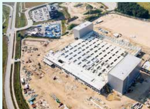
Northvolt Dwa Construction November 2022
